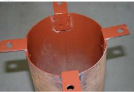
Next, duct tape all exposed bolts and place the pier and cap on a painting tarp. Apply an even coat of primer.
