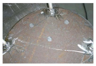
Place the tip of the wire welder at the edge of the hole and weld the bolt to the edge.
