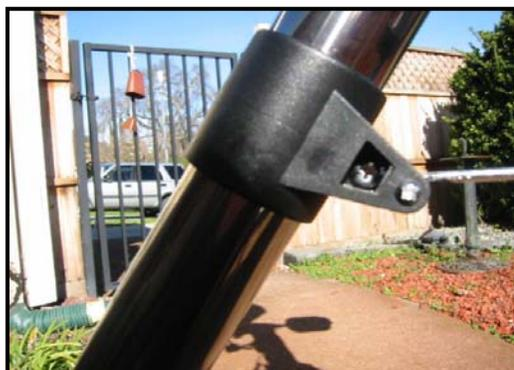
loosening the clamps and moving them upward, you can achieve the proper angle for stability.
